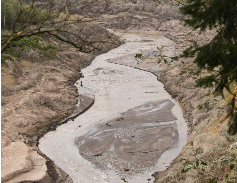
Figure 14. Photo of White River at Mud Mountain Dam during the growing season showing vegetation immediately adjacent to the stream. Note extensive fine sediment input to river, sparse riparian vegetation, bare river banks and lack of any shade along the river channel. Photo by Scott Anderson, Washington Water Center: https://www.usgs.gov/media/images/white-river-mud-mountain-dam
